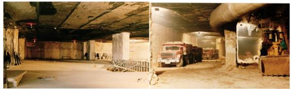
Figure 1. Kızılay station constructed by top-down construction method [2]
