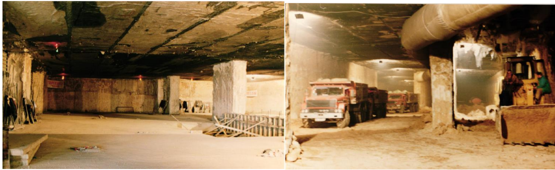
Figure 1. Kızılay station constructed by top-down construction method [2]
