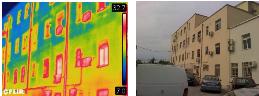
Figure 4. Image from thermal camera
