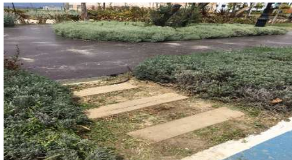
Figure 8. Floor covering (Original)
