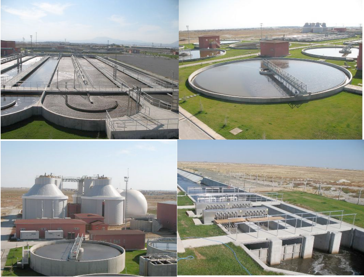
Figure 1. Konya WWTP general view and photos of the units
