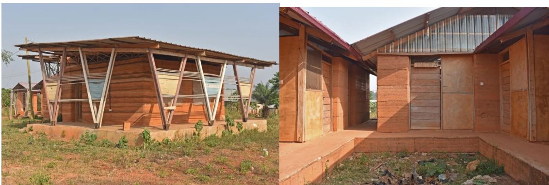
Figure 15. At Abetenim Arts Village, rammed earth and other modern earth-building techniques are promoted as a local and sustainable alternative to concrete blocks. These are practices run by the US-based non-profit Nka Foundation, which supplied local African youth with the opportunity to develop practical skills that will enable them to find employment in, the Republic of Ghana (Access 8).
